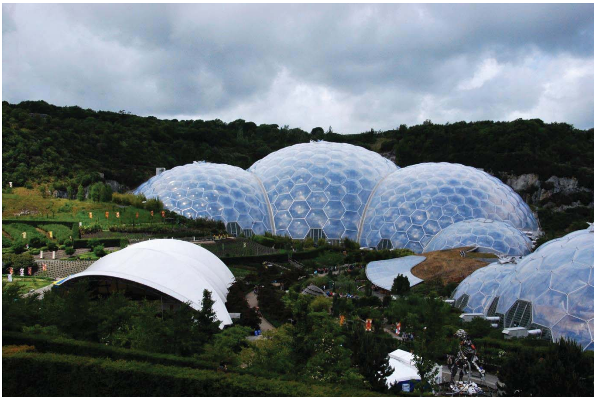
Figure 4 Eden Project Biomes, from Matthew Webb; personal collection; 18 Jun 2011.
